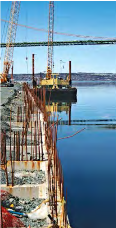
RICHMOND TERMINALS CONSTRUCTION
